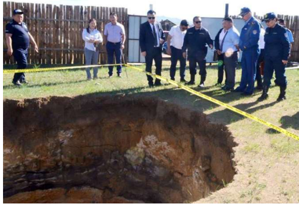
Figure 8. Thermokarst failure of the land of the city of Nalaykh
