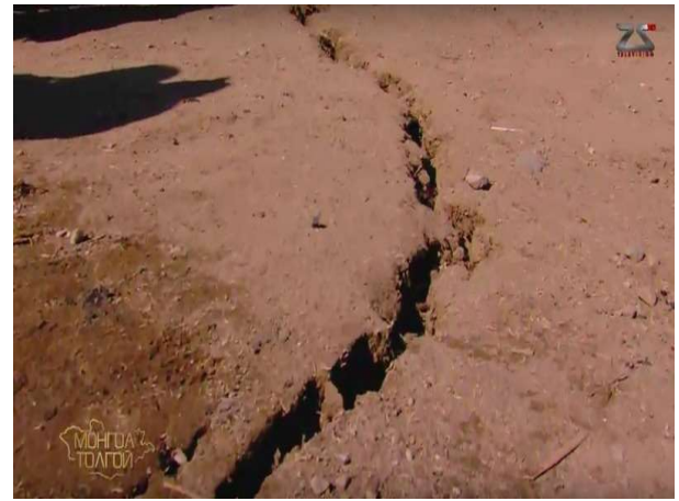
Figure 9. Crack in the ground of the city of Nalaih
