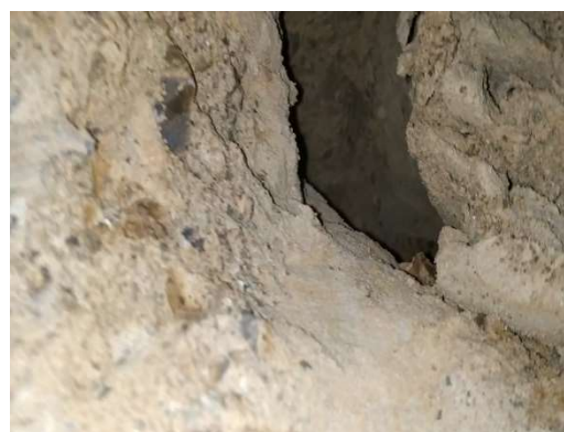
b - Well -11, at a depth of 7.35 m, direction from east and north;
