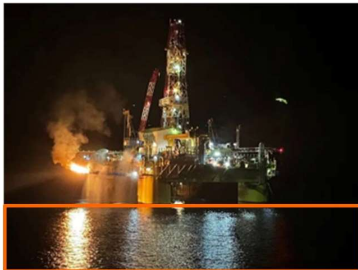
Fig. 21. Drilling platform "Offshore Oil 982" on the site of the Baodao 21-1 gas field [17].
