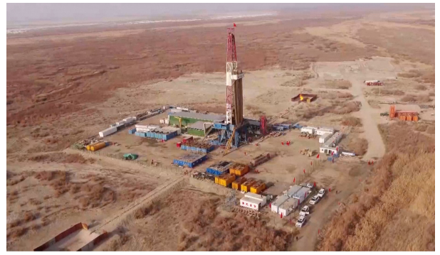
Fig. 12. Photograph of the drilling site of the Luntan-1 well [36].
