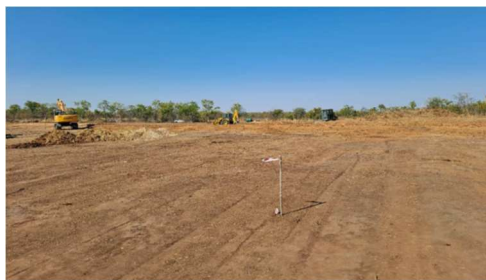
Fig. 8. Photograph of the Mukuyu-2 well drilling site [1].
