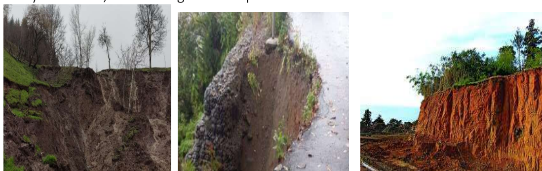
Figure 1.2.3. Adjara landslide (Kobuleti)
