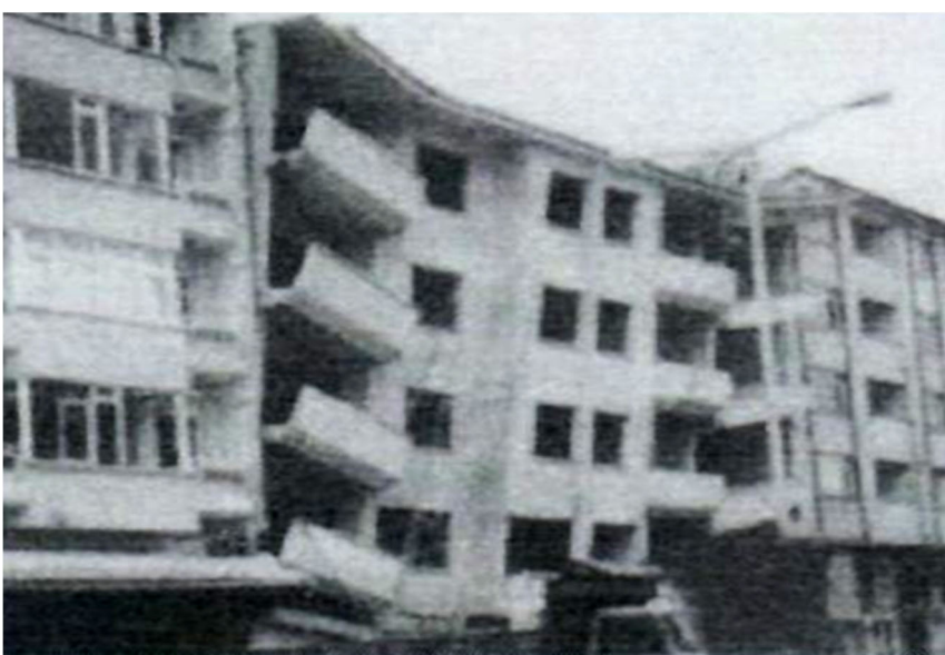
Fig.3 Hammering Effect
