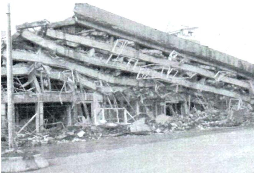
Fig.2 Strong Beam-Weak Column failures
