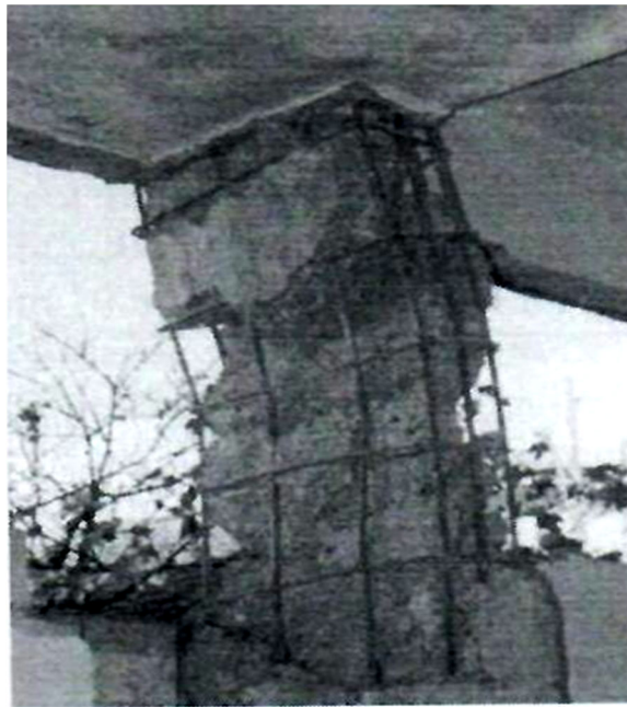
Fig.4 Short Column effect and failure
